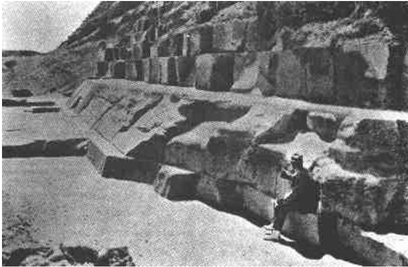
Figure 3.7 - Casing stones that still exist along the base perimeter of the Great Pyramid.
